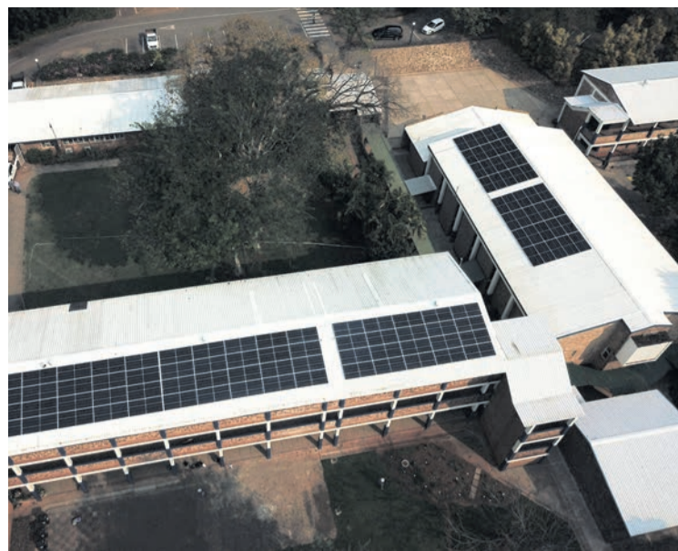
The layout of the solar panels on the roof at Unicorn Preparatory School. > Photos: Supplied
