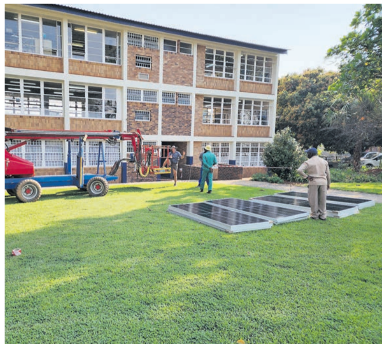
Installation of the solar system at Unicorn Preparatory School.
